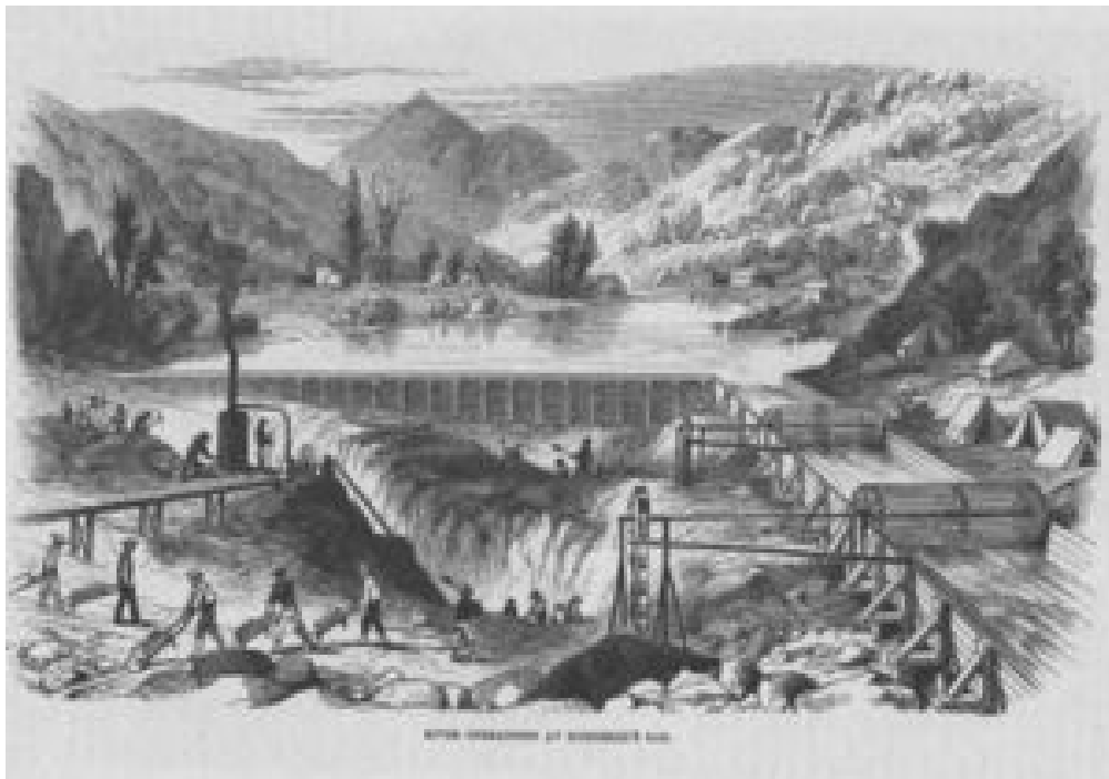
Gold miners excavate a river bed after the water has been diverted into a sluice alongside the river.
