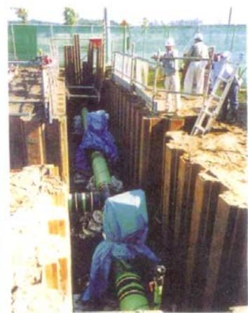
Photo 1 Application example of self-standing type steel sheet pile wall
