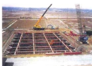
Photo 2 Application example of strut-type earth-retaining wall
