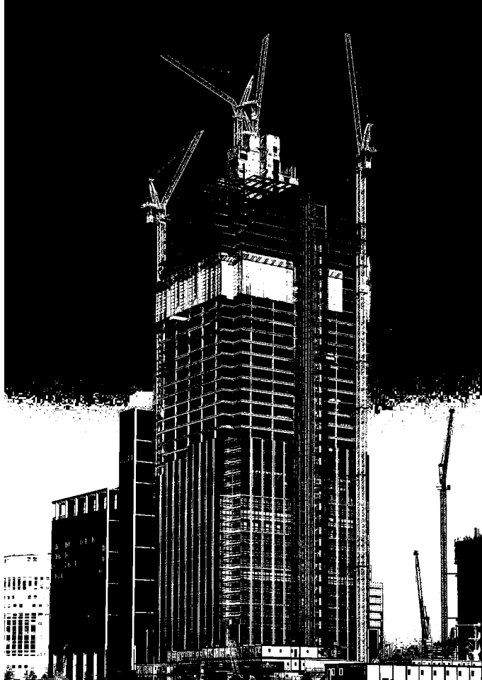
Fig. 33.12 Citigroup Tower, London showing tower cranes tied into the building (courtesy of Victor-Buyck Hollandia)
