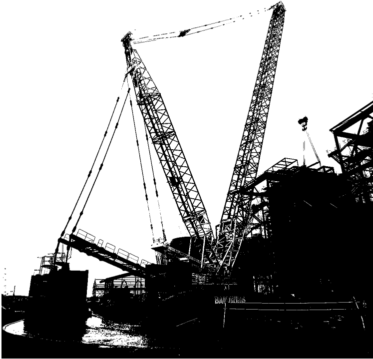
Fig. 33.8 Crawler crane (courtesy of Baldwin Industrial Services/Chapman Brown Photography)
