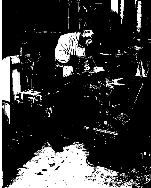
Fig. 24.7 Manual metal-arc welding of structural components (Photograph courtesy of The Lincoln Electric Company)
