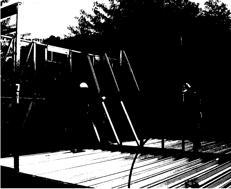
Fig. 5.30 Light steel framing using prefabricated panels
