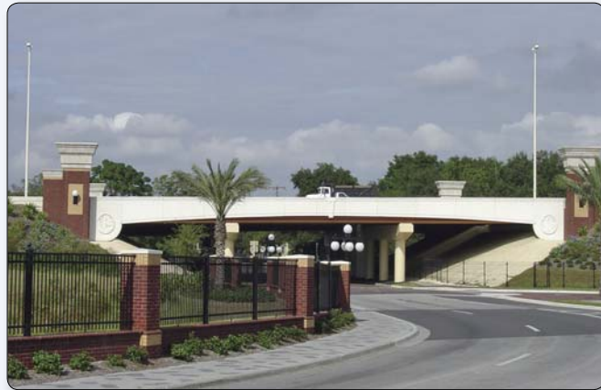
Figure C.18 – A variety of monumental decorative treatments have been added to this interstate overpass to disguise a standard-design bridge and attempt to make it compatible with a nearby brick factory and associated workers' housing historic district. Treatments like this should be avoided.
