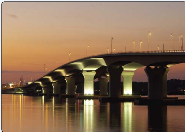
Figure C.20 – The Hathaway Bridge is located in Panama City, Florida. The structure is a variable depth segment bridge built in balanced cantilever. The pier-up lighting illuminates the piers and the underside of the superstructure. The designers chose to light the piers on either side of the navigation channel and only the ends of the side piers.
