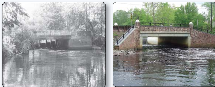
Figure D.20 – This box beam bridge, which relies on applied decoration instead of good aesthetic design for its appearance, illustrates what can happen when historic context is not understood. Built in an area where native stone is not common and thus not used for bridge superstructures and parapets, this bridge, with its retarditaire detailing, ignores the fact that the steel stringer historic bridge it replaced was a straight-forward example of up-to-date technology when it was built in 1914. The result is a pretentious design that is not compatible with the actual history and character of the proto-industrial 19th and early-20th century town. Designs like this should be avoided.
