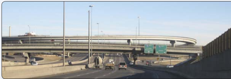
Figure C.4 – This multi-level system interchange uses a common superstructure type to visually unify a complex geometry. I-25 and I-70 Interchange, Denver, Colorado.
