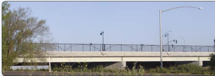
Figure C.12 – Decorative fencing was utilized on this bridge over I-80 in Davis, California to create a community gateway. A simple arched pipe attachment to the fence echoed the relief on the exterior parapet face. The strong silhouette of the fencing is memorable, yet relatively inexpensive to construct.
