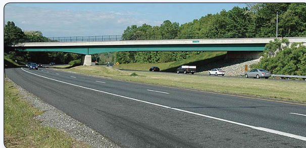
Figure D.4 – A well-chosen green can help a bridge fit a wooded background. This example would be improved by choosing a green closer in hue to the foliage behind it. I-83, Maryland.
