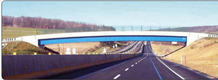
Figure D.13 – Contrast in color brings out the arched vertical profile of this overpass. Pennsylvania Turnpike near Somerset.
