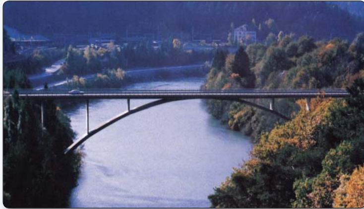
Figure B.3 – Rock foundations permit arch bridges. Reichenau Bridge, Switzerland.
