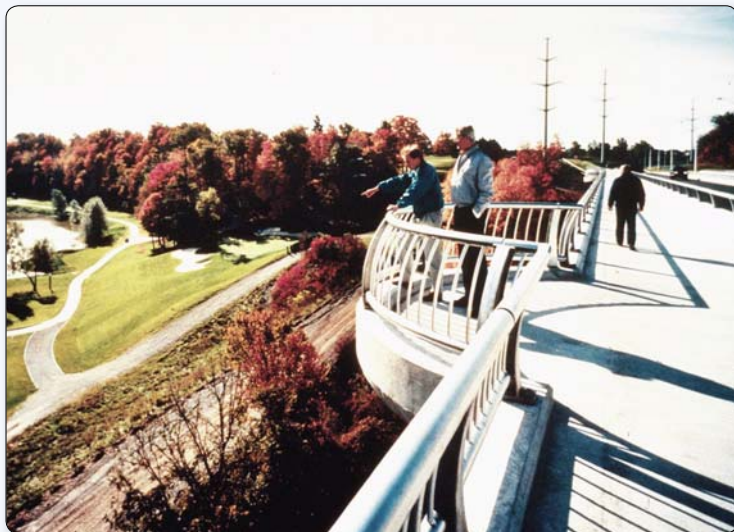
Figure B.4 – Having pedestrians on a bridge suggests the addition of overlooks. Upper Middle Road over 16 Mile Creek, Oakville, Ontario.
