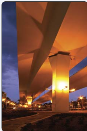
Figure C.22 – The S.E. 17 th Street Causeway Bridge is located in Ft. Lauderdale Florida. The approach spans are variable depth segmental built in balanced cantilever. The feature lighting was installed on the approach spans as well as the bascule span. The fixtures illuminate the pier columns and the bottom of the superstructure.
