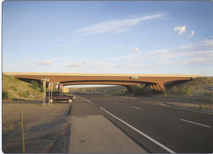
Figure C.17 – An excellent application of color was used to blend this slant leg frame concrete bridge into the high desert landscape. I-25 over State Route 599, Santa Fe, New Mexico.
