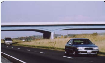
Figure D.2 – The haunch gives the girder a more interesting and attractive shape than a girder with parallel edges. It also indicates how the girder works structurally; it makes the girder deepest over the pier where the moments are the highest. I-81, Virginia.
