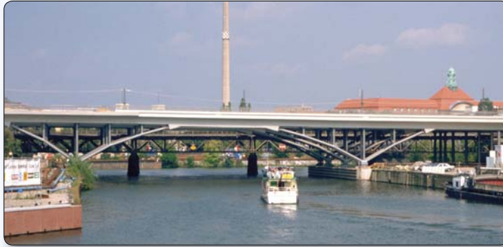
Figure B.5 – Marine channels and riverbank uses often affect bridge clearance requirements. Deutsch Bahn Railroad over Humbolthaven, Berlin, Germany.
