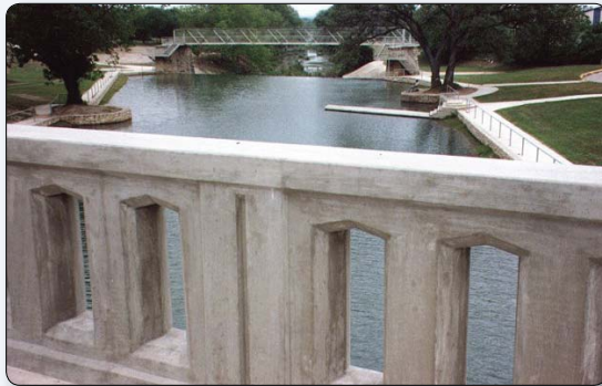
Figure C.10 – This crash tested railing is relatively transparent.
