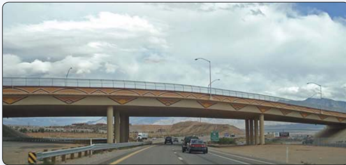
Figure D.1b – The lines of this decorative pattern criss-cross the parapet overhang line and muddy the clarity of the structure.
