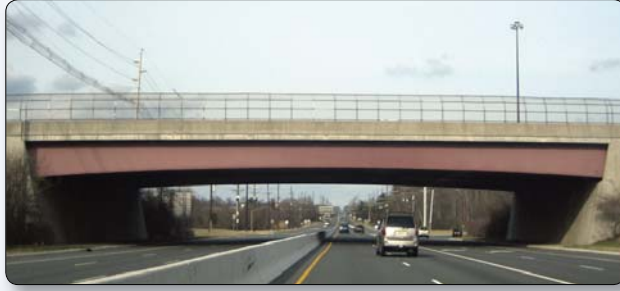
Figure C.3 – This bridge utilizes a haunched girder design with battered abutments to create an attractive span. The center median pier was eliminated to frame the view beyond the bridge and provide a gateway opening into the adjacent development. College Road over Route US 1, Princeton, New Jersey.
