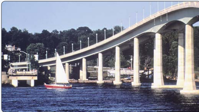
Figure D.10 – The larger main span creates a variation in the major rhythm of the piers, while the light posts create a consistent minor rhythm. Severn River Bridge (U.S. Naval Academy Bridge), Annapolis, Maryland.
