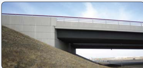
Figure C.7 – This mid-height abutment with a six-foot front face height eliminates the “sliver” silhouette of a stub abutment with a minimal abutment face height. E-470 standard bridge abutment, Denver, Colorado.
