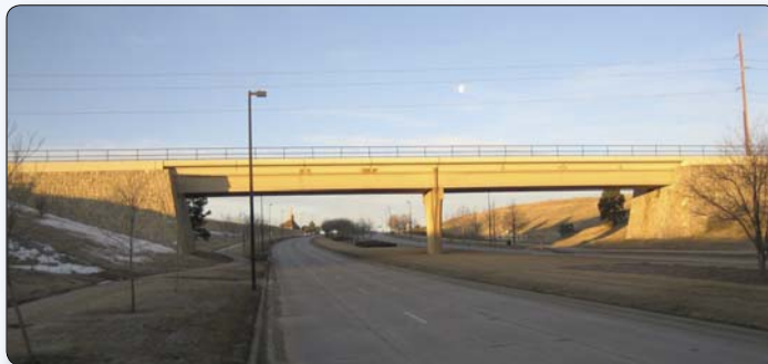
Figure B.8 – This community entry is in a depressed roadway section and passes under a bridge. The use of massive abutments combines with the roadway side slopes to form a gateway. Meadows Parkway Railroad Overpass, Castle Rock, Colorado.
