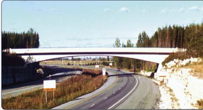
Figure D.9 – The proportions of this bridge, the large depth at the abutments compared to the depth at the crown, give it a very slender appearance. Ottawa, Canada.
