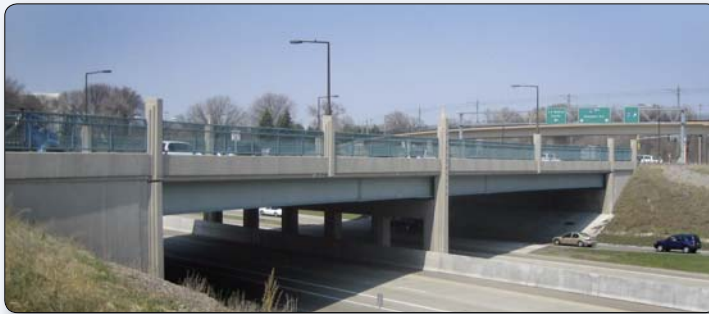
Figure C.13 – Columns have been placed at the outside edges of the pier cap, which emphasizes the vertical lines of the substructure. Similar corner details at the abutments strongly frame the bridge opening. Hiawatha Avenue over State Route 55, Minneapolis, Minnesota.
