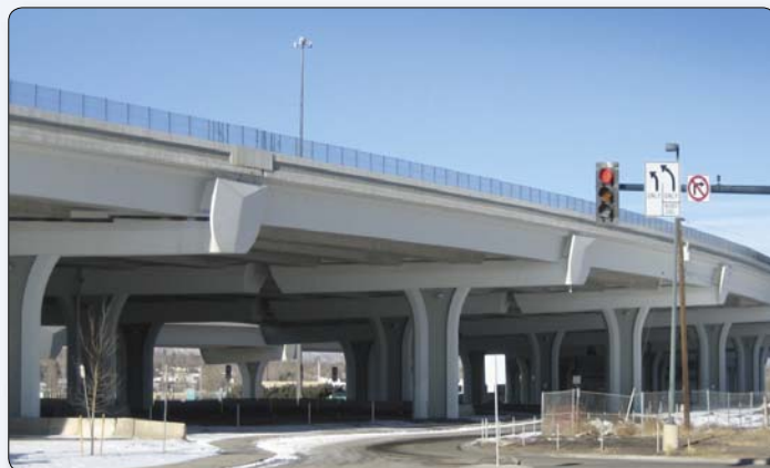
Figure C.1 – Wide bridges that are relatively close to grade often create visual barriers. In this case, use of post-tensioned caps increased the transparency of the substructure when viewed from an oblique angle. I-25 over Broadway Viaduct, Denver, Colorado.
