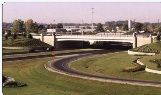
Figure D.12 – Freeway compositions work best when they are balanced about the median centerline. Avery Road over US 33, Dublin, Ohio.
