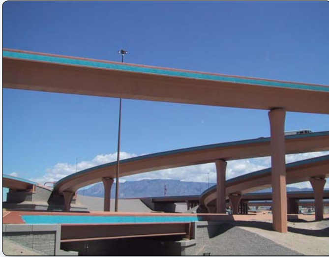
Figure B.9 – Albuquerque’s Big I interchange has a theme covering MSE walls, standard details and colors developed with community input.
