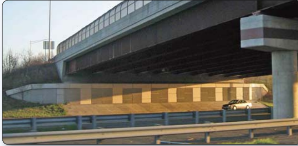
Figure D.5 – Using form liner patterns to create texture on an abutment wall. Scotch Road over I-95, New Jersey.
