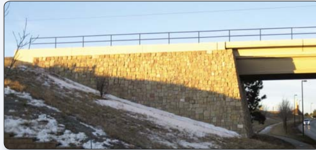
Figure C.8 – This full-height abutment strongly defines the ends of the bridge and acts as a gateway. BNSF Railroad over Meadows Parkway, Castle Rock, Colorado.
