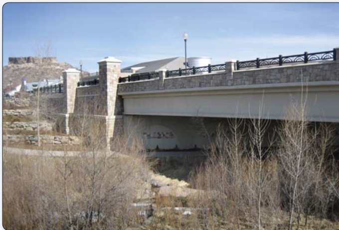
Figure C.16 – Pilasters and offset wall planes are used to break up the retaining wall surface and strongly define the ends of the bridge. This bridge is in a town park, and a monumental image was desired. Perry Street Bridge, Castle Rock, Colorado.
