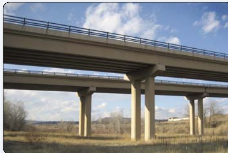
Figure C.6 – The substructure for this high level crossing with slender piers is virtually transparent. Meadows Parkway over Plum Creek, Castle Rock, Colorado.
