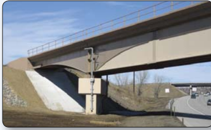
Figure C.19 – This drainage system and pier geometry clash with an otherwise attractive overall aesthetic scheme. Union Pacific Railroad Bridge over I-25, Castle Rock, Colorado.
