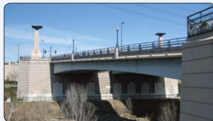
Figure C.14 – This haunched Steel box girder bridge carrying 20 th Street over the South Platte River in Denver, Colorado was designed as a gateway structure. The battered faces and rusticated surfaces of the full-height abutments add interest to this structure.
