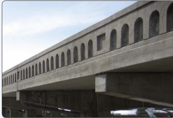
Figure C.11 – This deep barrier relief on a reconstructed concrete arch bridge is visually compatible with the original concrete barrier. State Highway 83 Bridge over Castlewood Canyon, Colorado.
