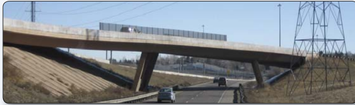
Figure C.2 – This bridge has a reverse superelevation between the abutments. The effect of this deck geometry is that the bridge appears to be twisted, drooping between supports, and varies in depth. It is doubtful that this is the aesthetic effect the designer intended. Ramp bridge at I-25 and I-225 Interchange, Denver, Colorado.
