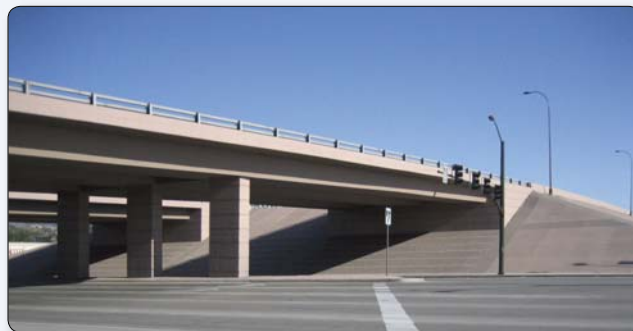
Figure C.9 – The shadow of the long deck overhang and relatively transparent barrier creates strong horizontal lines on this bridge. The superstructure appears to be very slender. I-25 over Woodman Road, Colorado Springs, Colorado.
