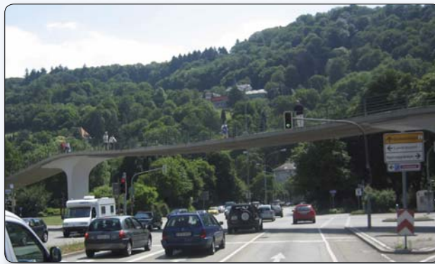
Figure D.18 – This stress ribbon bridge located in Freiburg, Germany provides a much-needed pedestrian crossing over a busy street. The bridge exhibits an excellent, economical design and has become a noteworthy structure in the community.
