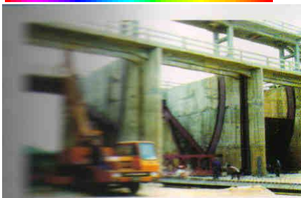
Valve gate of spillway
