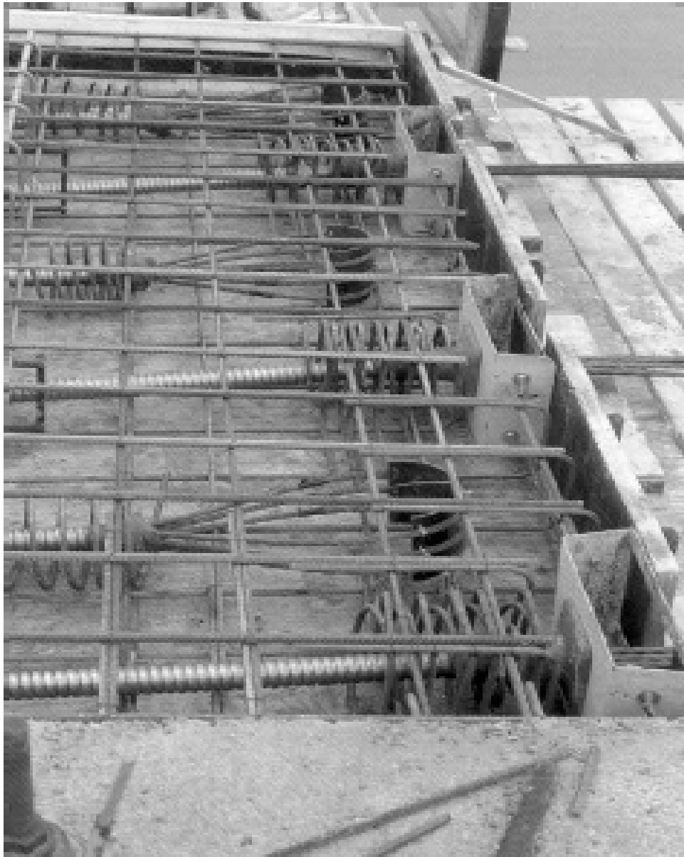
Figure 1.7: Anchorages provide for the safe introduction of post-tensioning forces into the concrete.
