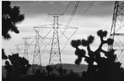
Figure 2 A \pm 500 -kV HVDC transmission line
