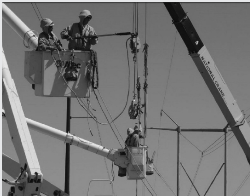
Figure 4 Re-conductoring a 345-kV line.
